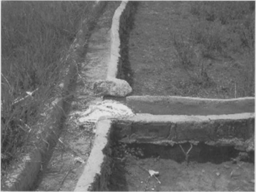
Fig. 9. — Irrigation canals constructed to carry the water from reservoir to cultivated fields.
