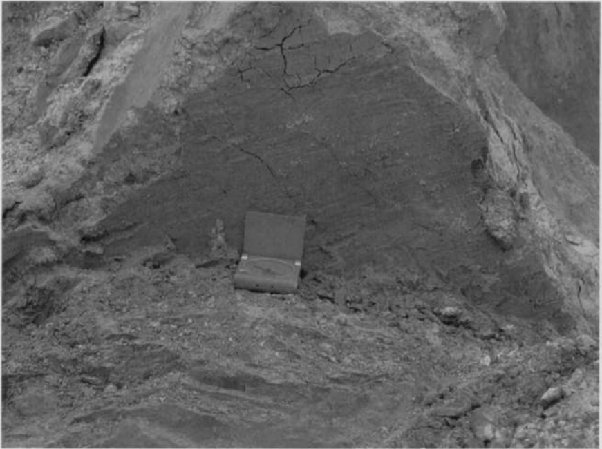
Fig. 6. — Slickenside on active fault observed in weathering cover of Neocene sediments, 6 km SE of Lao Cai city.
