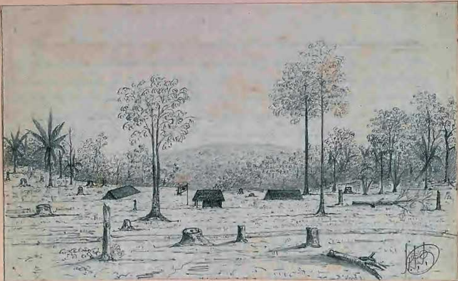
'Xkula Mando' clearing for Station
